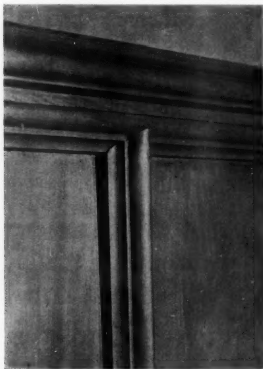
EFFECT OF UNEQUAL SHRINKAGE OF BUILT-UP RED GUM MOULDINGS
