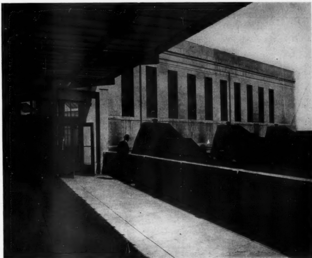
VIEW SHOWING STAIRS TO THE TRAIN PLATFORMS
