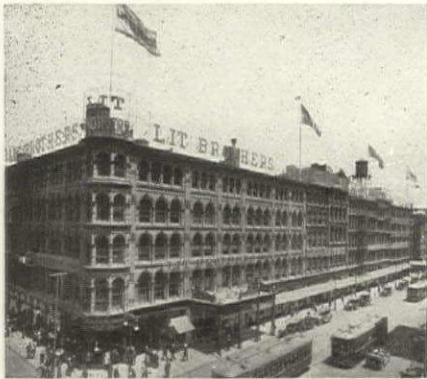
Lit Bros. Department Store, Philadelphia, Pa., is ventilated and freshened with ozonated air.
