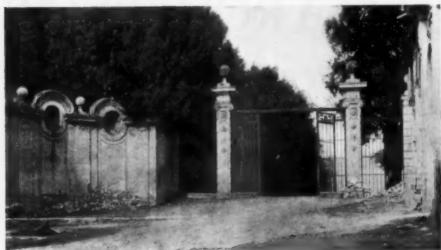
INNER GATEWAY LEADING TO CASINO TERRACE
