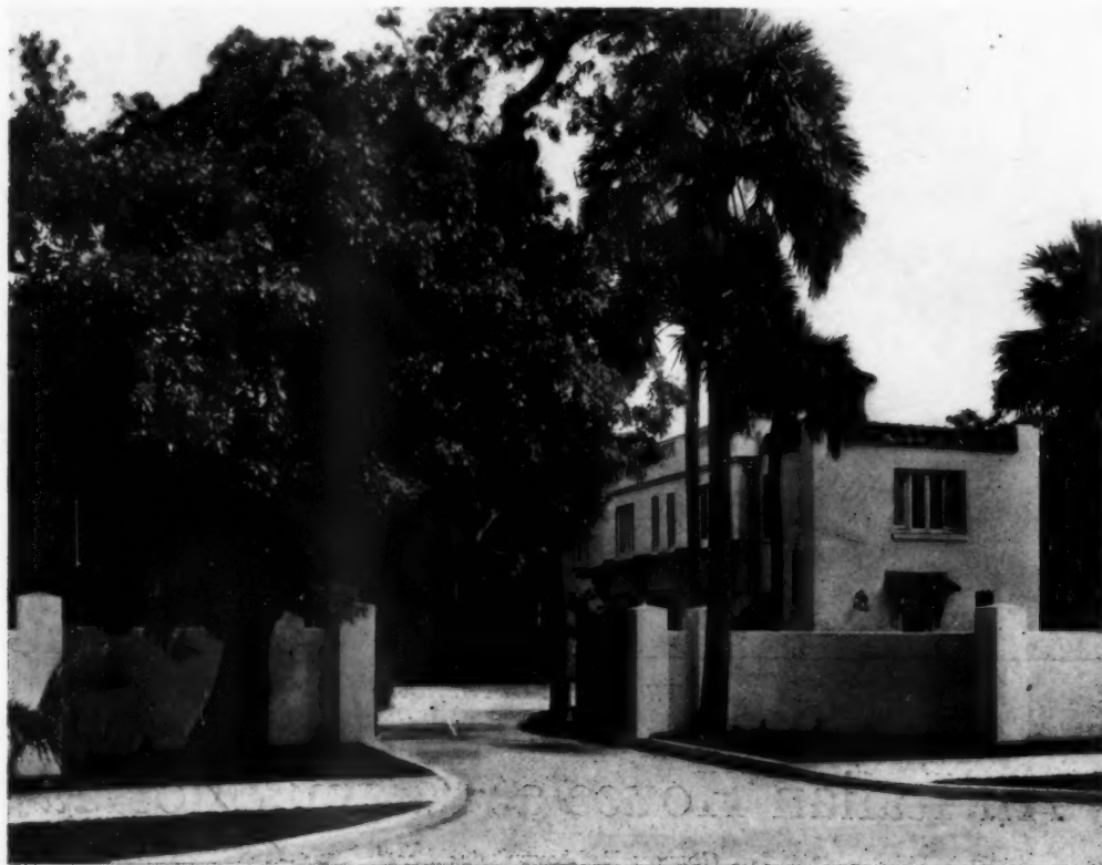
MAIN ENTRANCE AND GARAGE
