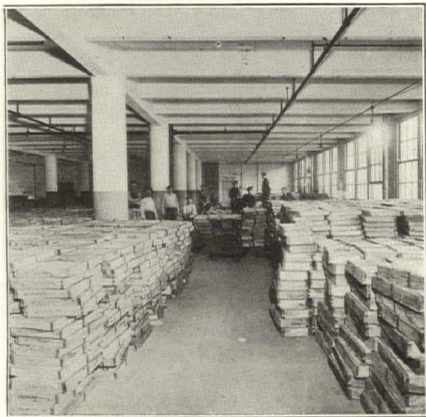
Interior view of second story showing heavy overload of tin. The work of removal has just been commenced.
