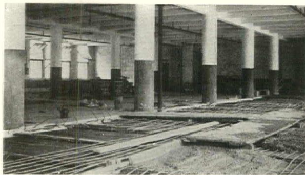
New slab being placed. Reinforcing rods showing are those taken out of demolished floor slab, straightened and re-used.
