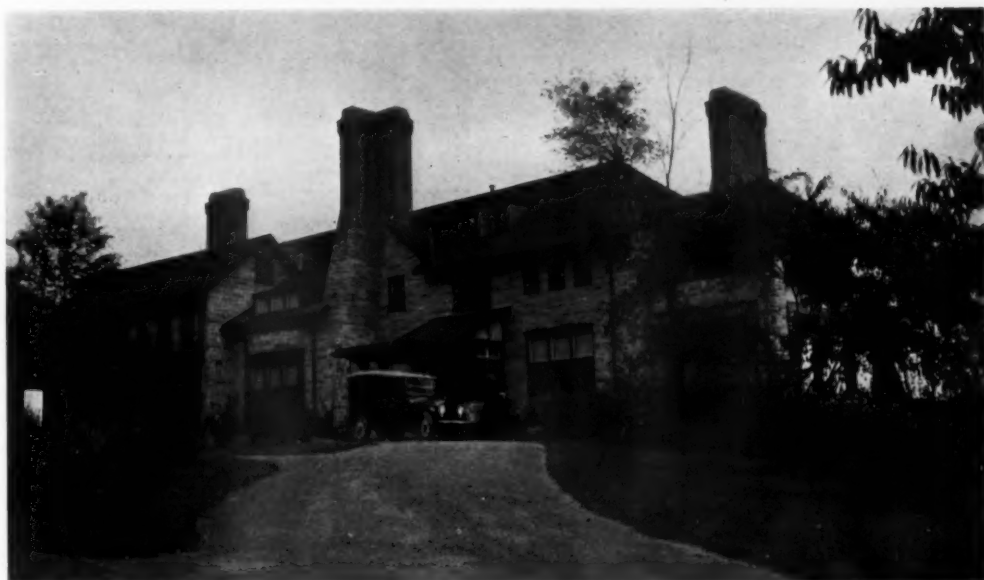
PHOTO 10. MAIN DRIVE AT JUNCTION WITH ENTRANCE TURN
