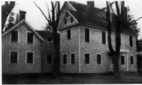
HOUSE BEFORE ALTERATIONS
