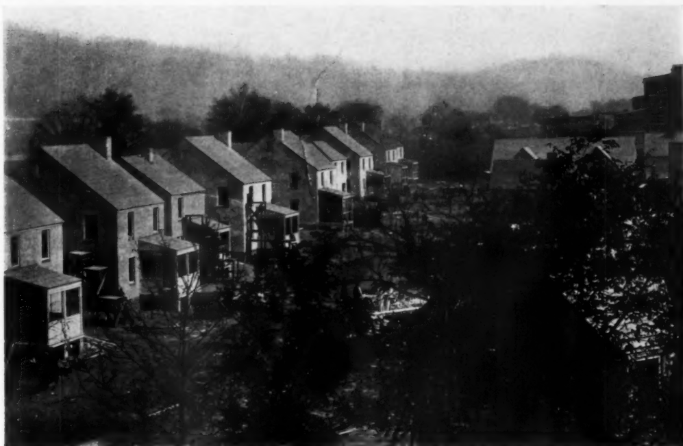
REAR OF HOUSES ON STREET NO. 5
