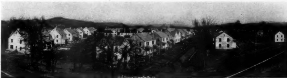
PANORAMIC VIEW, LOOKING EAST
