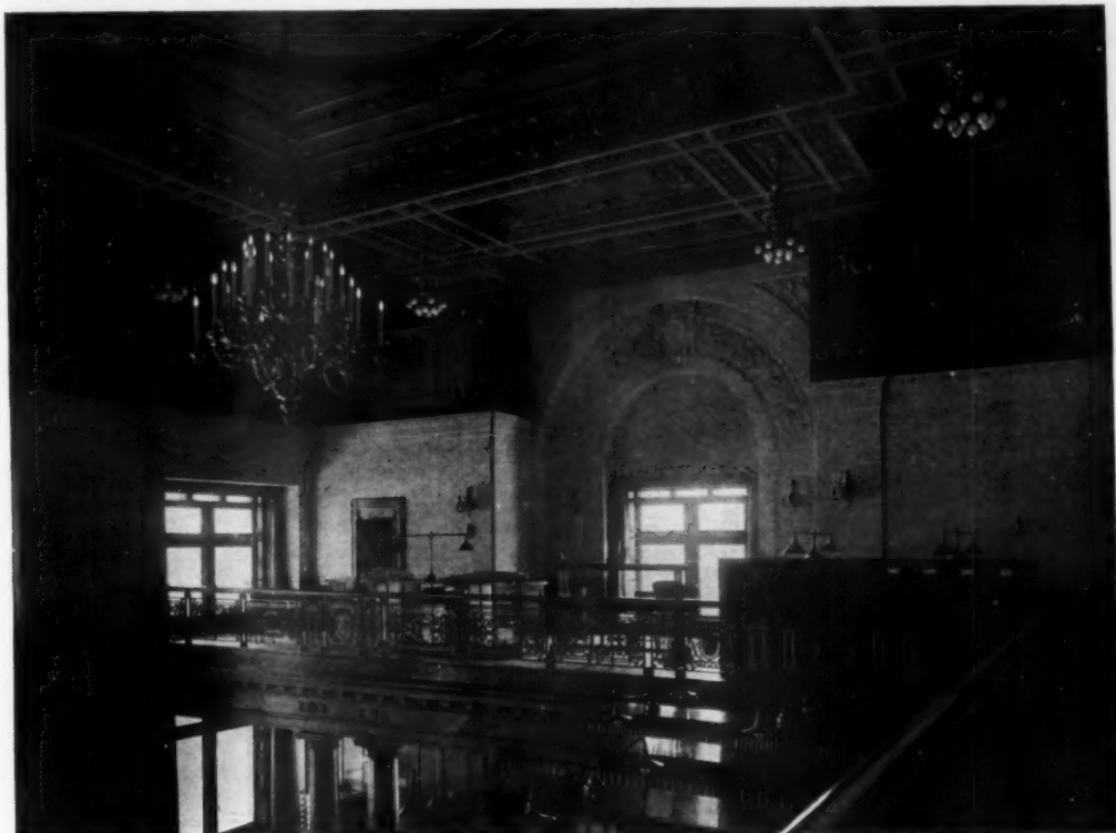
PLASTER CEILING, CONNECTICUT STATE LIBRARY, HARTFORD
