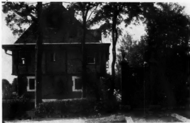
NORTH ELEVATION AND GATE, RABBIT HOUSE
