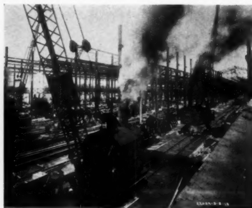
Erecting frame with locomotive cranes.
