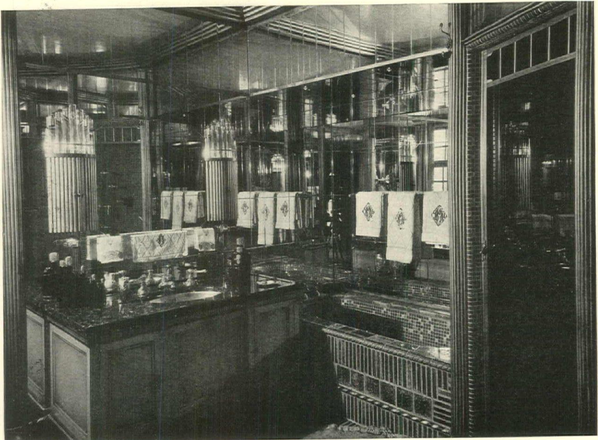
Photo by Gottscho
