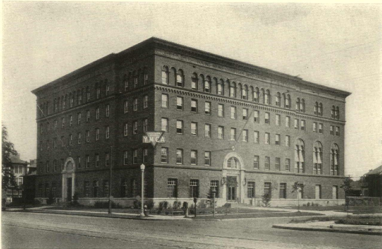
GENERAL VIEW OF EXTERIOR
