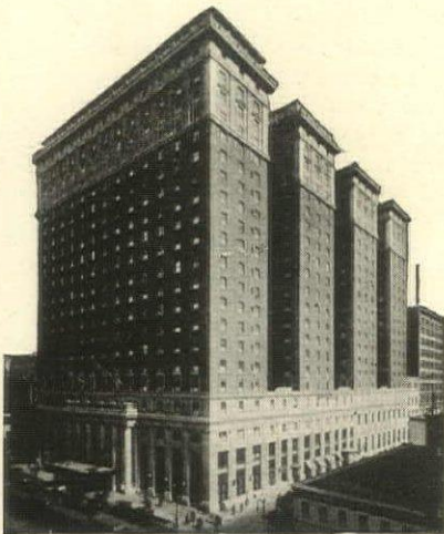
Every demand for hot water in the Hotel Pennsylv- vania is supplied by Whitlock Heaters.
