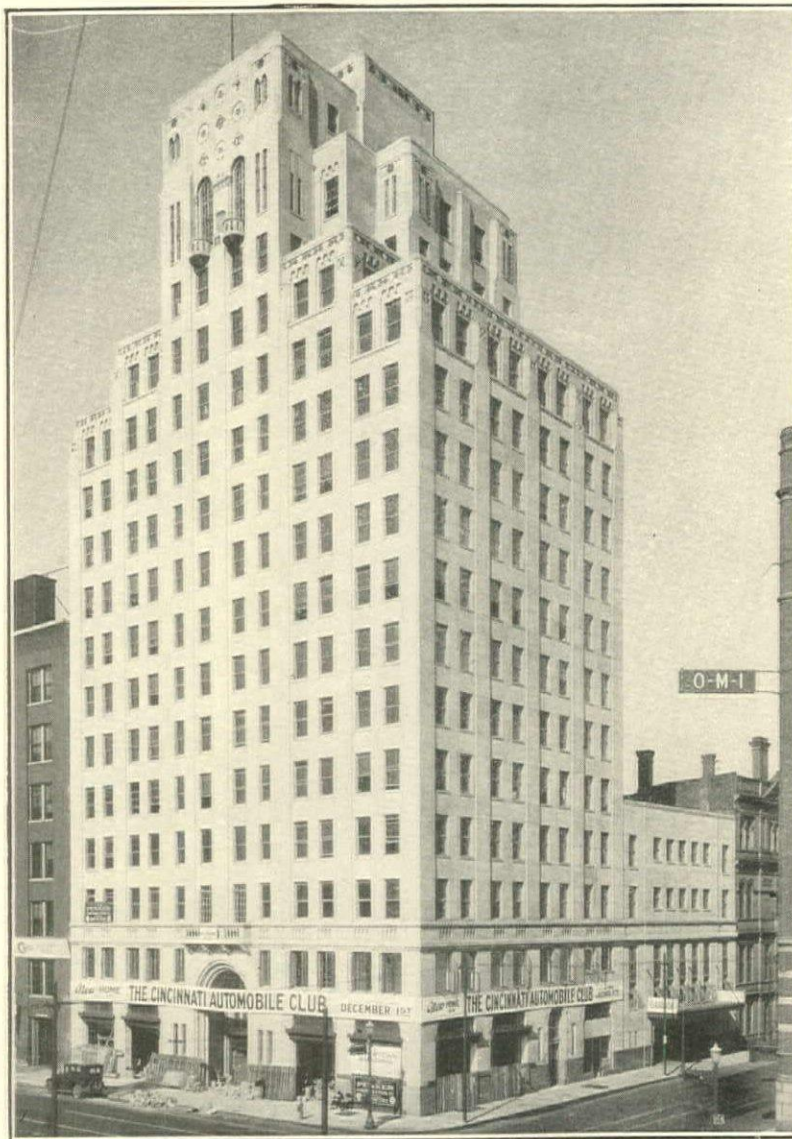
American Druggist Fire Insurance Co. Building, Cincinnati, Ohio. Joseph Steinkamp & Brother, Architects. Max Penker Sons Co., Builders. Variegated Indiana Limestone.
