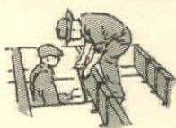
Hanging ceiling slabs
