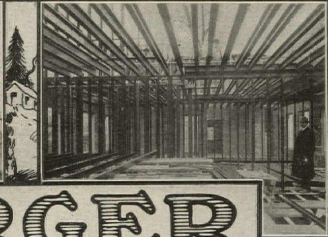
CONSTRUCTION VIEW - MR. BROMAN'S RESIDENCE. TOLEDO, O.
