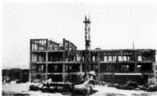
Building 1 under construction.
