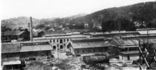
View northwest of Building 1, showing adjoining plant. A typical plant with low buildings, partially combustible and spread out for protection. No special provision for paved roads and economical intra-plant traffic.
