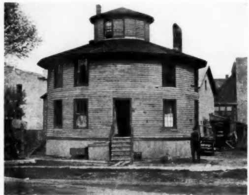
THE OLD ROUND HOUSE. BUILT IN 1836 Wood Siding on Concrete Walls
