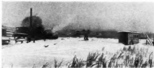
Site of the improvement on December 19, 1916.
