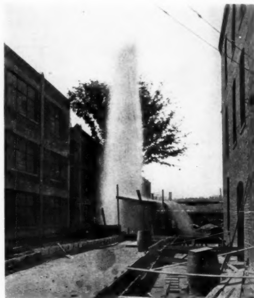
Shooting the brine well, 40 seconds after firing 120 quarts of nitro-glycerine. Well 1050 ft. deep, 8 in. diameter.
