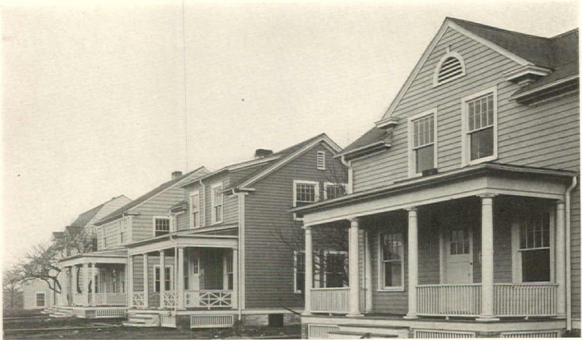
Maniwoc, Wis. E. F. Miller, Architect. 100 houses and 1 dormitory. Started Aug. 1, 1918; photograph taken Dec. 15, 1918. Houses completed.
