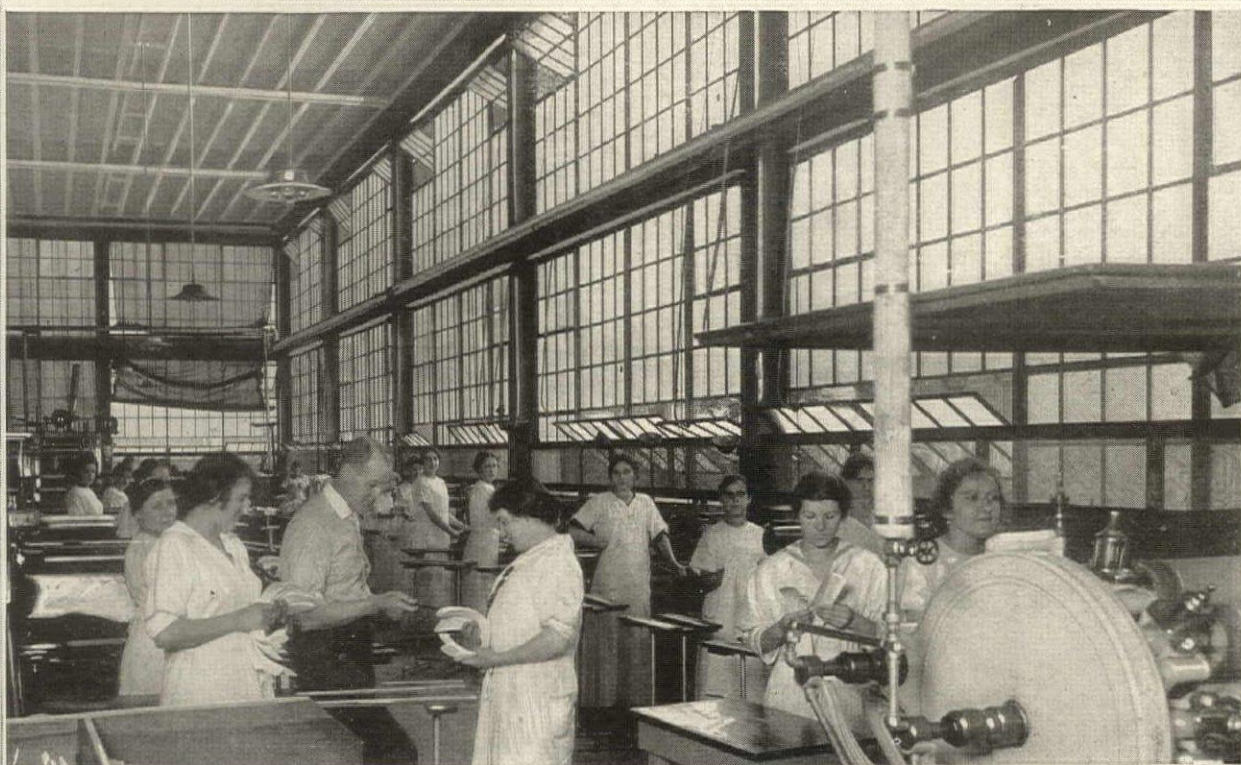
The Banner Laundry, Detroit, is designed along modern lines. Fenestra Solid Steel Windows are used to assure proper daylighting and ventilation, as explained below.
