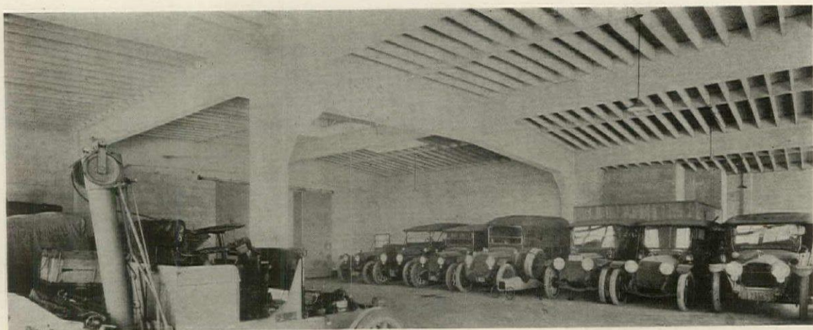
The second floor of the building on the N. W. corner of Second East Street and Social Hall Avenue. This floor is designed for the storage of motor trucks. The construction is of the rigid frame type discussed in the text.
