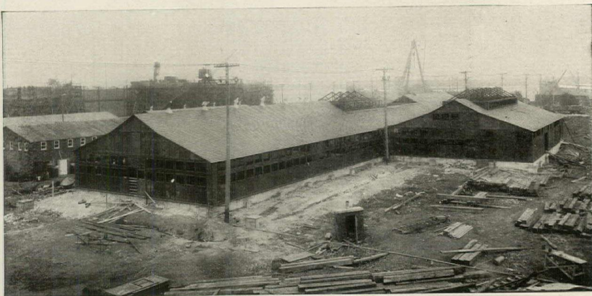
Construction of large dining hall and kitchen at Great Lakes Engineering Works, Ecorse, Mich. Smith, Hinchman & Grylls, Architects and Engineers, Detroit, had complete charge of the planning, details, construction and arrangement of these Truscon Steel Buildings.
