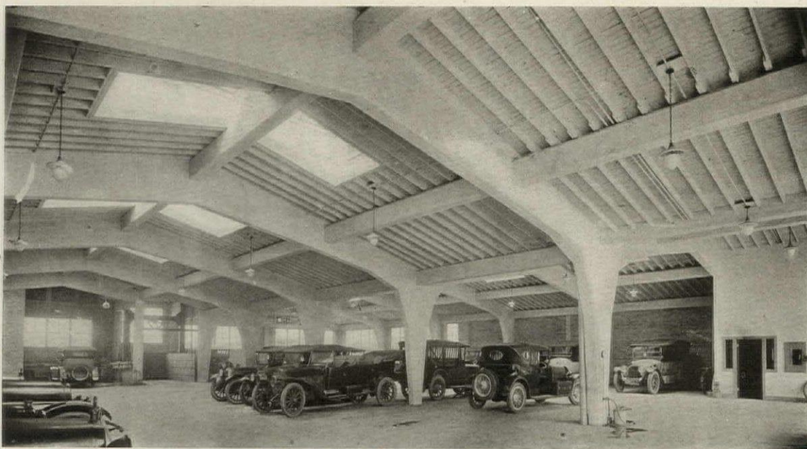
An interior view of the Social Hall Avenue Garage, showing the rigid frame type of reinforced concrete construction.
