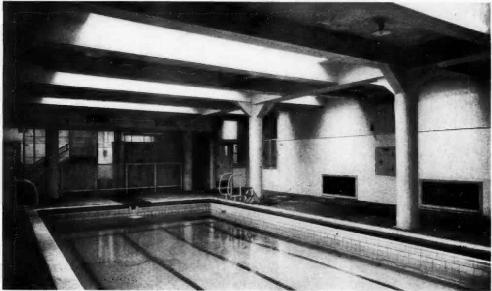
Fig. 7. General view of the pool and natatorium facilities in Public School No. 66, Borough of Brooklyn. The plan of this pool is shown in Fig. 2. Note the guide lines on the floor of the pool, also the generous register openings for fresh air supply and ventilation.
