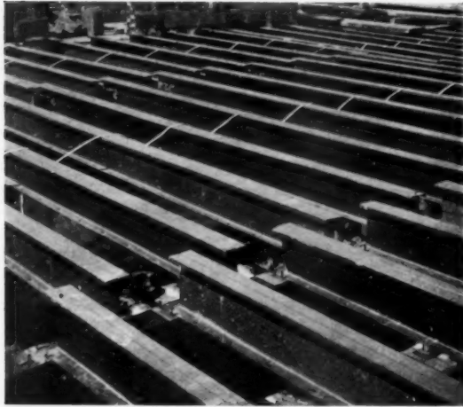
Floor construction in a large apartment house, metal joists supported on structural steel girders, galvanized iron bridging strips in place.
