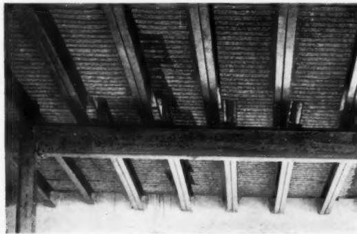
A floor with metal joists, structural steel girders and columns. Concrete floor slab in place. View from below.
