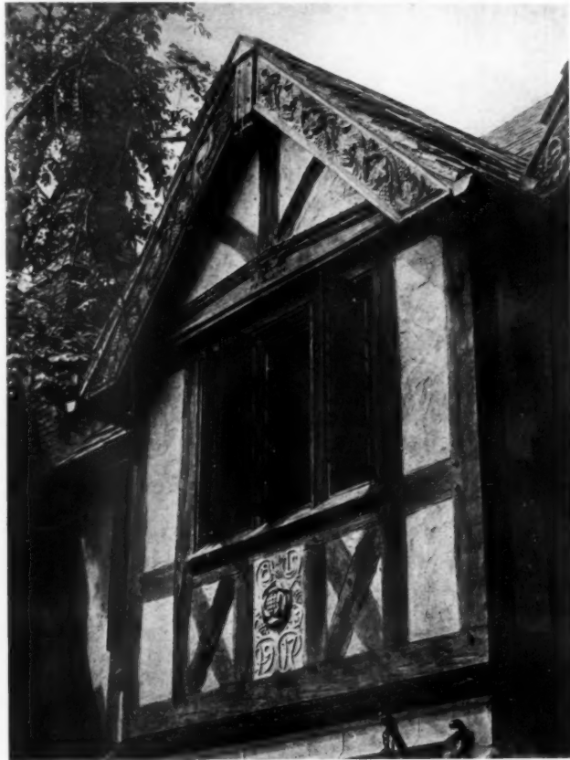
DETAIL OF GABLE OVER ENTRANCE
