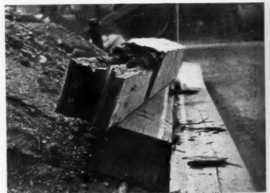
Fig. 19. Beam rotted for some distance from column, serving as rain water conductor, which it enclosed.
