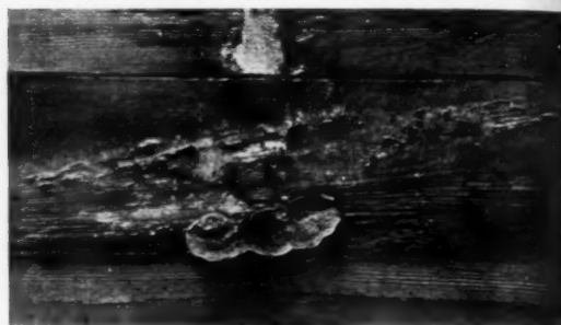
Fig. 4. Fruiting plants of Lenzites Seperia growing on southern pine roof planks of a cotton mill weave-shed after the sheathing was removed for some time. They are of a brown color.
