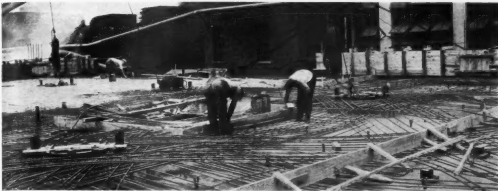
View of a partially poured concrete floor, showing the four-way reinforcing rods in place
