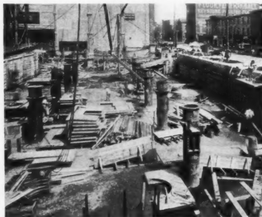
Basement columns in position with slab form material ready for erection
