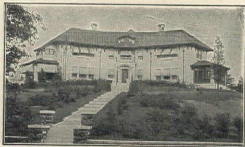
Stained with Cabot's Stucco Stains
