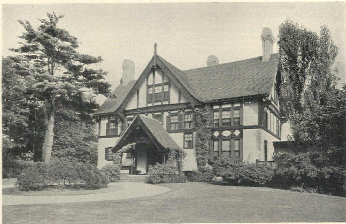
HOUSE OF L. H. H. JOHNSON, MILTON, MASS. COOLIDGE & CARLSON, ARCHITECTS
