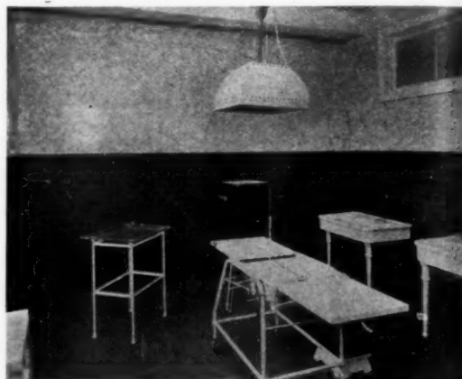
Fig. 14. Special operating room of St. Joseph's Hospital, Stockton, California. Thomas Mulcahy, Architect.
