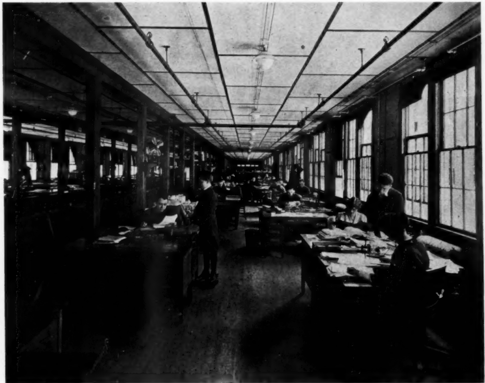
VIEW IN ONE OF THE BAYS IN THE UNITED STATES BUILDING FOR DIVISION OF MILITARY AERONAUTICS
