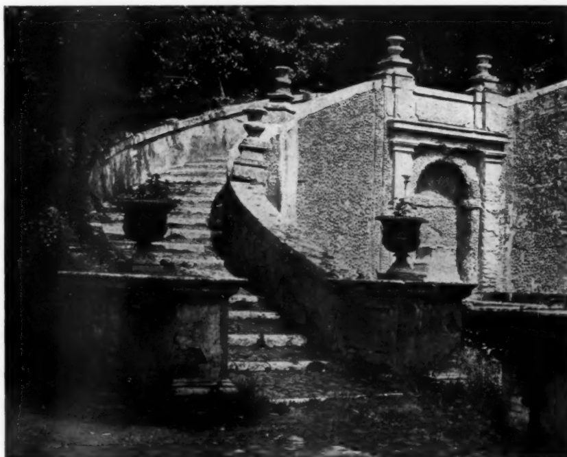
DETAIL OF STAIRWAY, GARDENS OF VILLA D'ESTE
