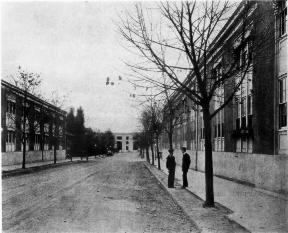
VIEW LOOKING NORTH ON EIGHTEENTH STREET, BETWEEN BUILDING FOR COUNCIL OF NATIONAL DEFENSE AND FUEL BUILDING No. 2
