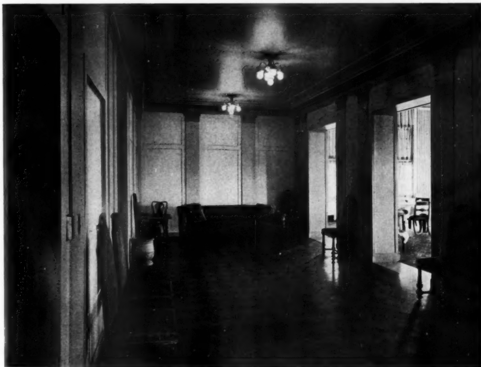
LOBBY TO MAIN DINING ROOM UNIVERSITY CLUB, ST. LOUIS, MO. EAMES & YOUNG, ARCHITECTS
