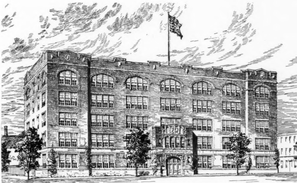
THE STANDARDIZED ELEMENTARY OR INTERMEDIATE SCHOOL BUILDING, NEW YORK
