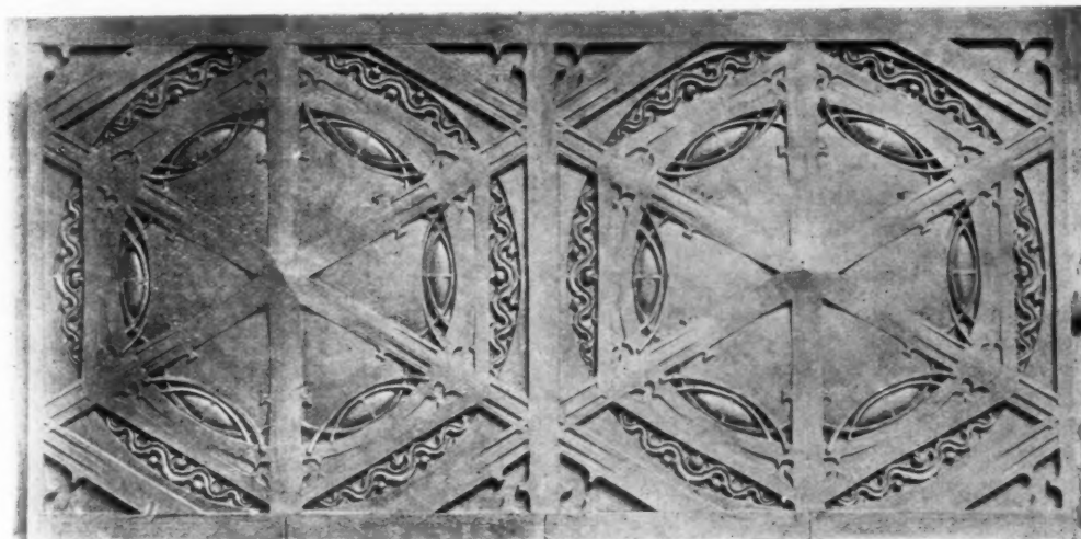
DETAIL OF PARAPET
