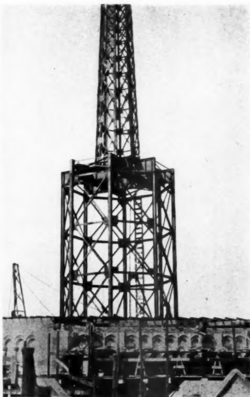
Fig. 14. The framework of the lantern and lower portion of the fleche.
