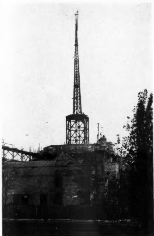
Fig. 19. The frame of the lantern and fleche completed. Placing the cross in position with a mast derrick. Construction trestle at the left.
