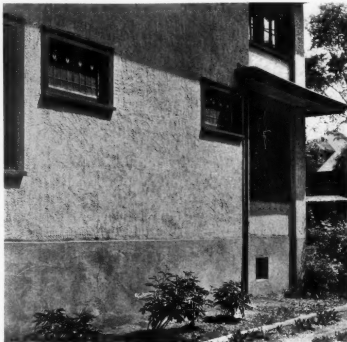
Photographed 36 months after completion. Magnesia cement stucco applied to wood lath and with a sponge-stippled finish. Note the color and texture of the work. The basement wall is of stone and finished with another material
