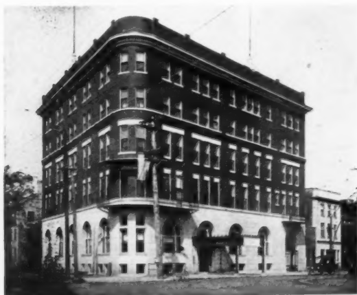
Magnesia cement stucco applied to the first story of a brick hotel in lieu of stone
