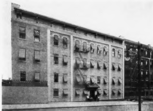
An old institutional building, in New York City, converted into apartments. Magnesia cement stucco applied to a brick wall that has been repeatedly painted
