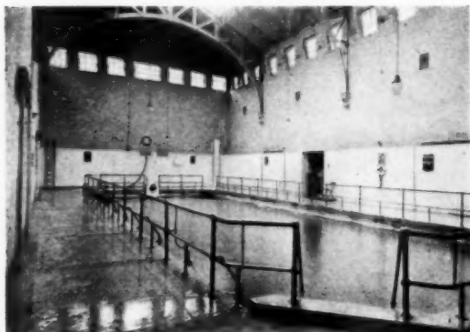
A view of the Twenty-third Street Swimming Pool. The upper part of the mixing tower is seen at the far end of the room.
