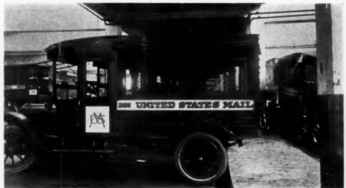
VIEW ON FIRST FLOOR. NOTE THE OVERHANG OF THE TRUCK OVER THE ISLAND PLATFORM SHOWING THE NECESSITY OF SUFFICIENT WIDTH FOR CLEARANCE FROM OPPOSITE TRUCKS
