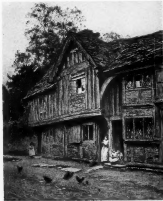
ROOF OF SLATE TILES, HALF TIMBERED, WITH BRICK NOGGING
