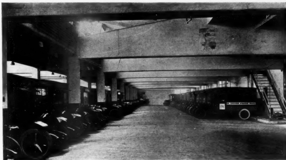
VIEW ON THE FIRST FLOOR. EXCELLENT DISTRIBUTION OF DAYLIGHT THROUGH THE SAWTOOTH SKYLIGHTS. NOTE OVERHANG OF THE TRUCKS OVER THE WALL PLATFORM AT THE RIGHT.
