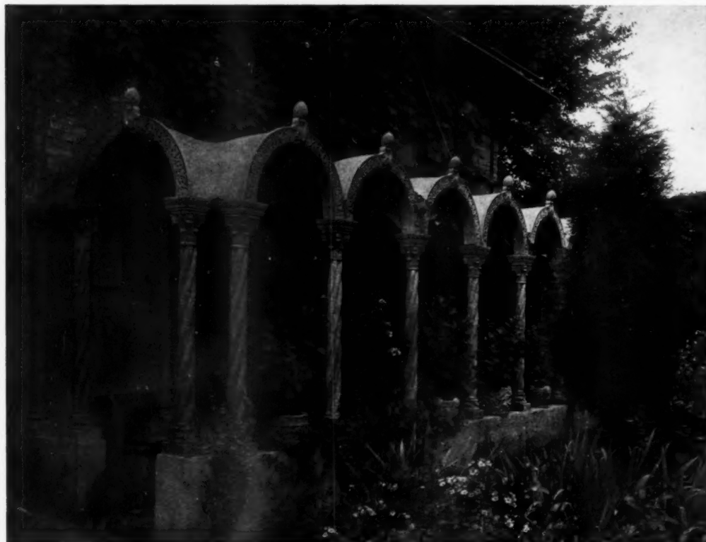
Delicate tracery such as ordinarily would be left to the stone cutter's art is readily molded in concrete. The more intricate patterns are reproduced by casting the material in glue molds. The units are afterward assembled just as is any other masonry.
