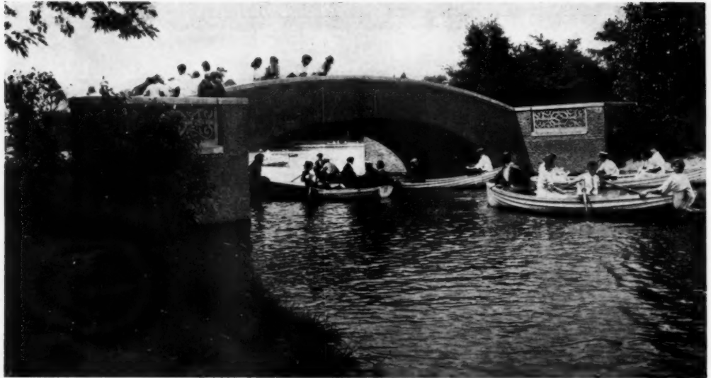
The decorative possibilities of concrete are combined here in the precast unit panels and the slap-dash surface finish.
