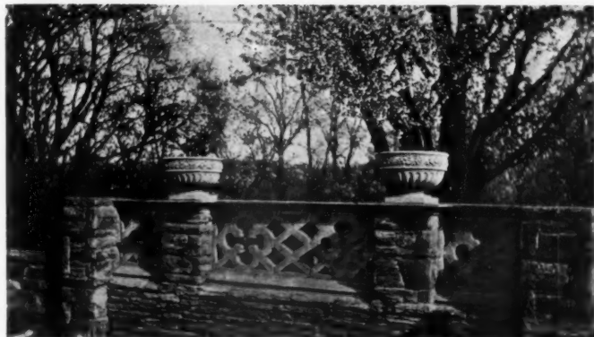
An example of irregular coursed stone masonry combined with precast concrete units to form a balustrade and the decorative features of it.
