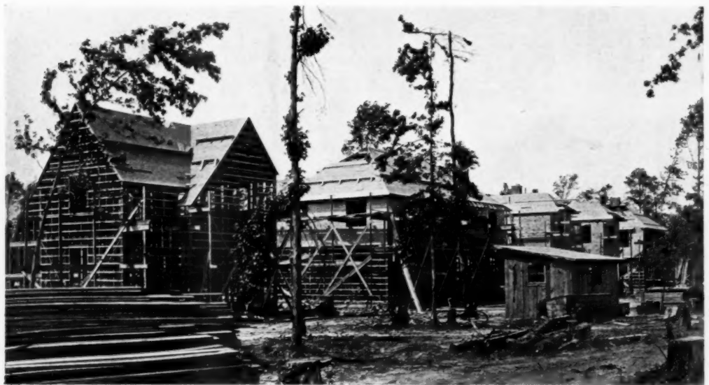
REAR VIEW OF ABOVE HOUSES
