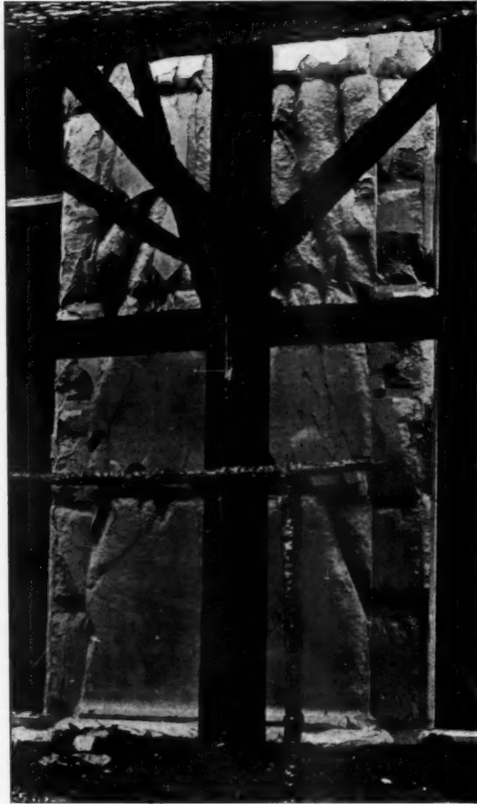
Fig. 3—View showing the spalling of the limestone veneering. Fourteen of these piers between windows and doors opposite the sidewalk protection were damaged
