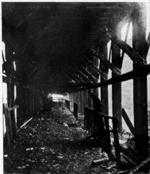
Fig. 2—Interior view of sidewalk protection. About midway between the walk and the underside of the material platform at the top may be seen a few remaining horizontal rafters of the rainshield over the walk. This shield and a sheathing at the side next the building were both of light boards and contributed chiefly to the rapid spread of the fire and the intense heat
