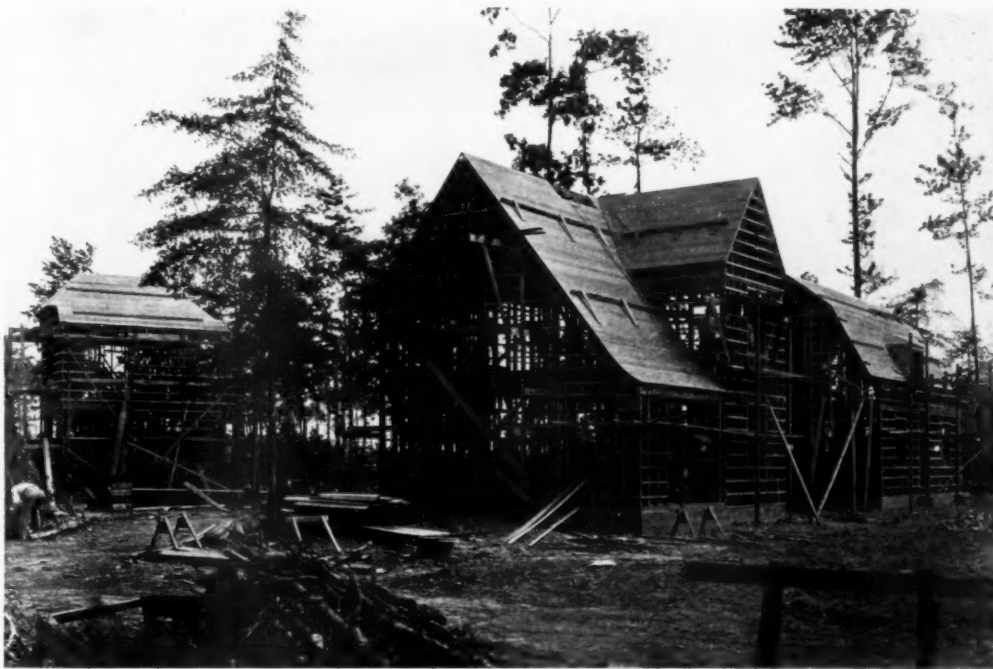
PROGRESS PHOTOGRAPHS OF HOUSES, TYPES E-1 and B-1
