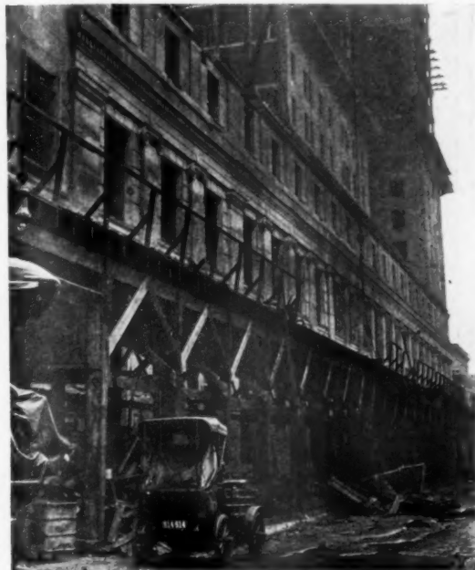
Fig. 1—West Thirty-third Street front of Pennsylvania Hotel, looking west, showing general view of building and sidewalk protection
