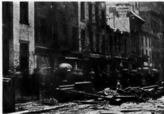
Fig. 5—View showing the damage by fire to wooden doors, window frames and cornices on the fronts of buildings across the street from the fire
