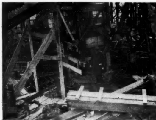
Compression ring at the crown of the main inner dome.
