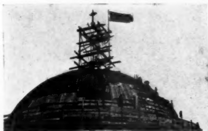
Constructing the main dome
