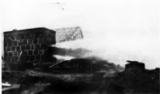
TEST VAULT IN ACTION
