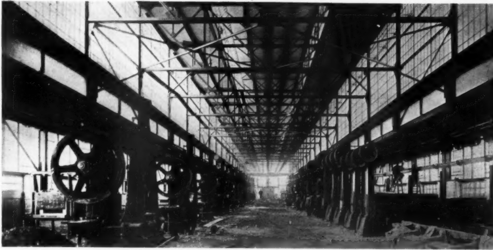
INTERIOR VIEW OF FORGE SHOP, PACKARD MOTOR CAR COMPANY, DETROIT ALBERT KAHN, ARCHITECT
