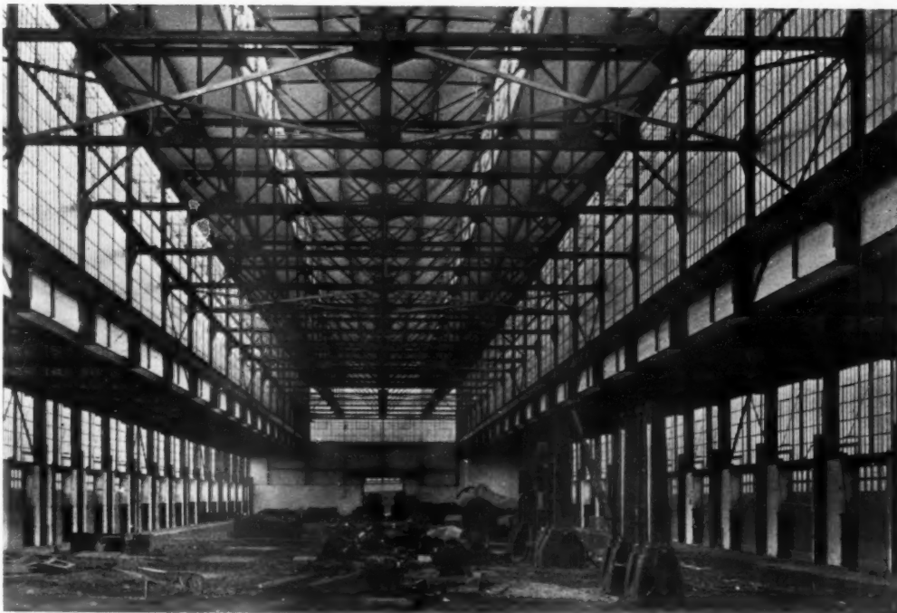
INTERIOR VIEW OF FORGE SHOP, PACKARD MOTOR CAR COMPANY, DETROIT ALBERT KAHN, ARCHITECT
