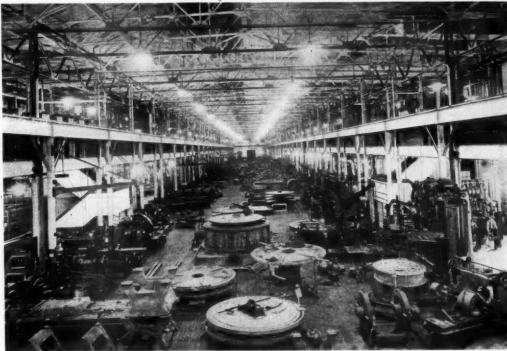
MACHINE AND ASSEMBLING SHOP WITH ARC LAMP INSTALLATION
