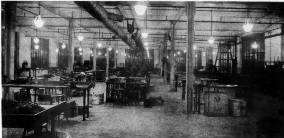
A SHOP WITH WHITE WALLS AND CEILING FOR SMALL MACHINE WORK, FINISHING AND ASSEMBLING
