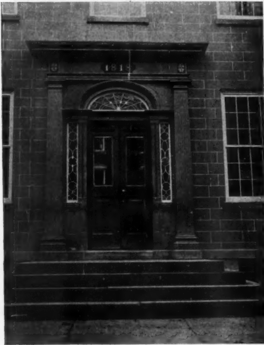
ENTRANCE TO COURT HOUSE The Original Doors Have Been Replaced
