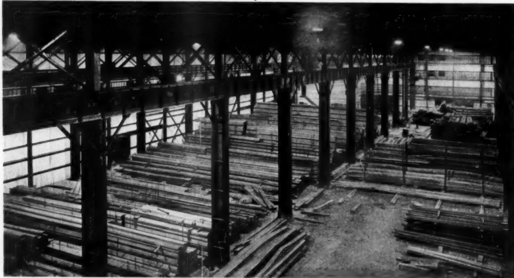
STOCK ROOM OF A METAL WORKING PLANT WITH WHITE WALLS.
