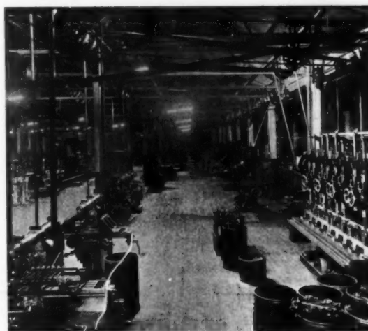
INSTALLATION OF MERCURY-VAPOR LIGHTING UNITS.
