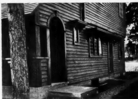
KITCHEN ENTRY IN SHARP PERSPECTIVE, SHOWING THE BEADED WEATHERBOARDS
