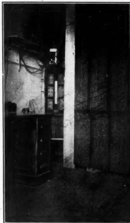
THE FRONT OF BOX COVERED AND READY FOR BLANK RUN TEST
