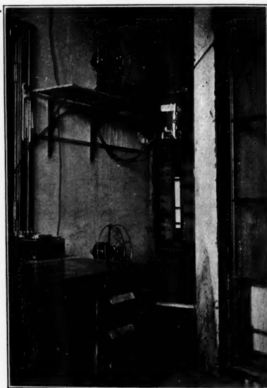
THE FANS, SWITCHBOARDS, METERS AND GENERAL ARRANGEMENTS
