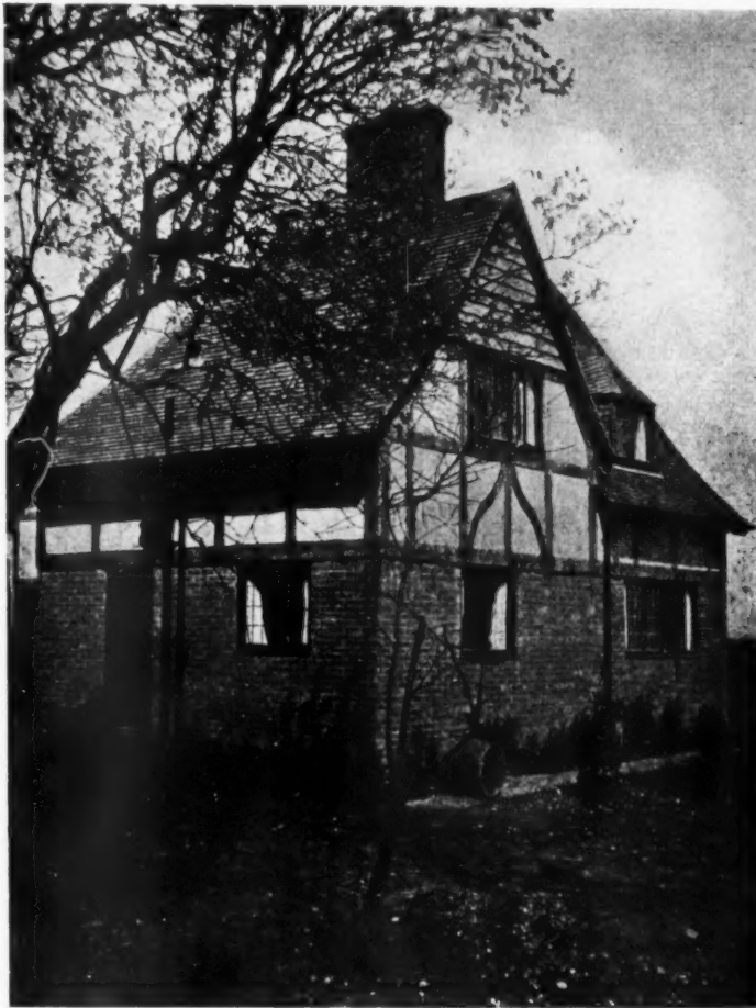
WORKINGMAN'S COTTAGE AT BEAULIEU, HAMPSHIRE.
