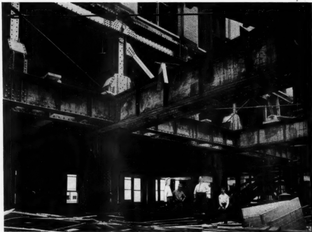
Figure 3. OLD TRUSSES REMOVED
