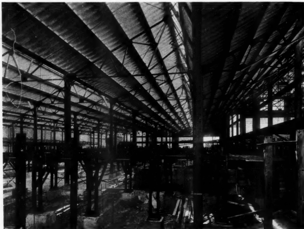
INTERIOR VIEW SHOWING GYPSUM ROOF SLABS IN PLACE WHITNEY GLASS COMPANY, GLASSBORO, N. J. THE DeVORE-McGORMLEY COMPANY, ARCHITECTS
