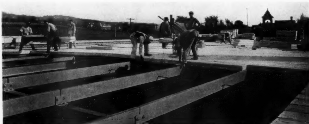
PLACING SLABS ON ROOF
