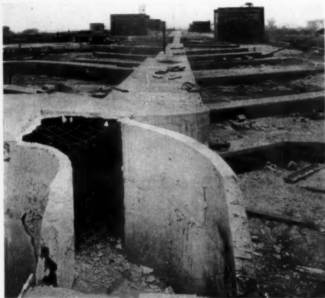
VENTILATING DUCTS ON ROOF, WITH REINFORCED GYPSUM CEILING AND CURVED SIDE WALLS POURED ON THE JOB. STRAIGHT WALLS MADE OF FACTORY CAST TILE WITH ONE SMOOTH FACE SAXON MOTOR COMPANY, DETROIT H. H. LANE, ARCHITECT
