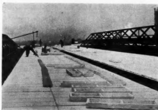
PLACING ROOF SLABS IN WINTER
