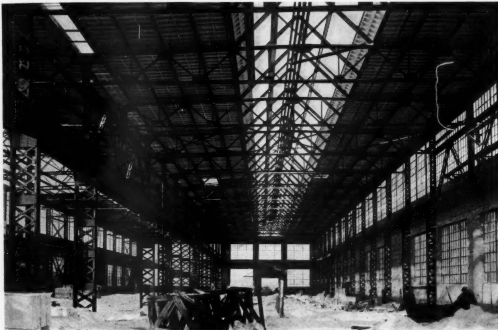
INTERIOR VIEW SHOWING GYPSUM ROOF SLABS IN PLACE AMERICAN SPIRAL PIPE WORKS, CHICAGO DAVIDSON AND WEISS, ARCHITECTS
