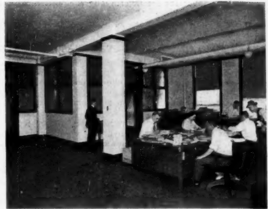
SHOP OFFICE—THE PYLE-NATIONAL COMPANY, CHICAGO
