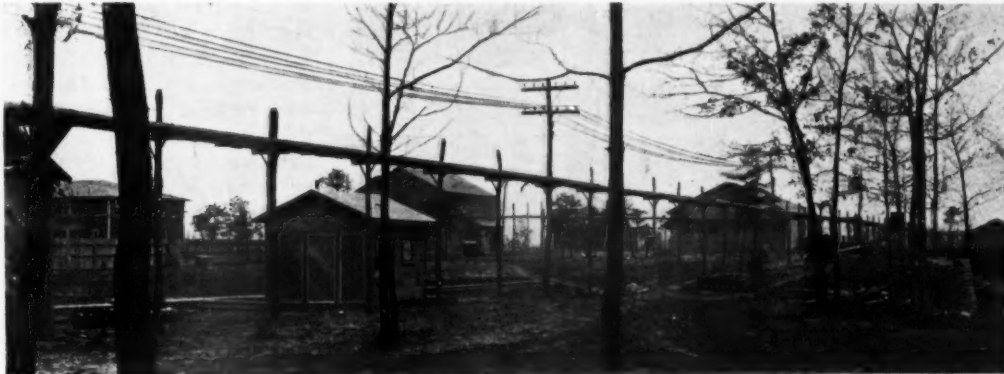
PLANT OF THE OLIVER LOADING COMPANY, OLD BRIDGE, NEW JERSEY
