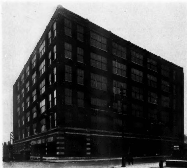
BUILDING FOR THE WILLYS-OVERLAND COMPANY, SAINT LOUIS MILLS, RHINES, BELLMAN AND NORDHOFF, ARCHITECTS
