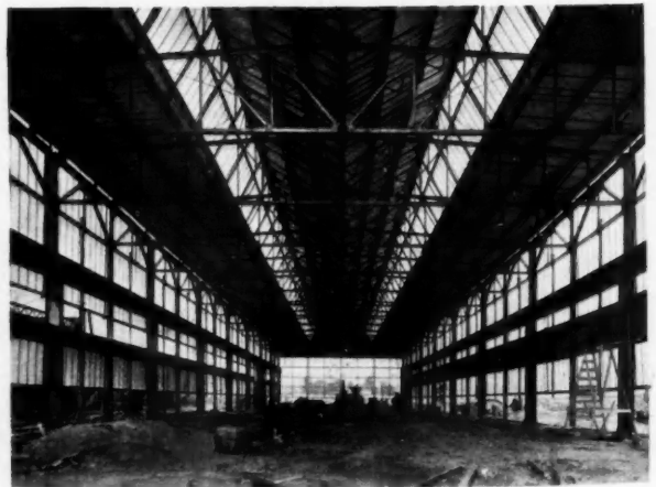
SHOP WITH BOTH SIDE AND ROOF LIGHTING. BUILDING OF HYDRAULIC PRESSED STEEL CO.
