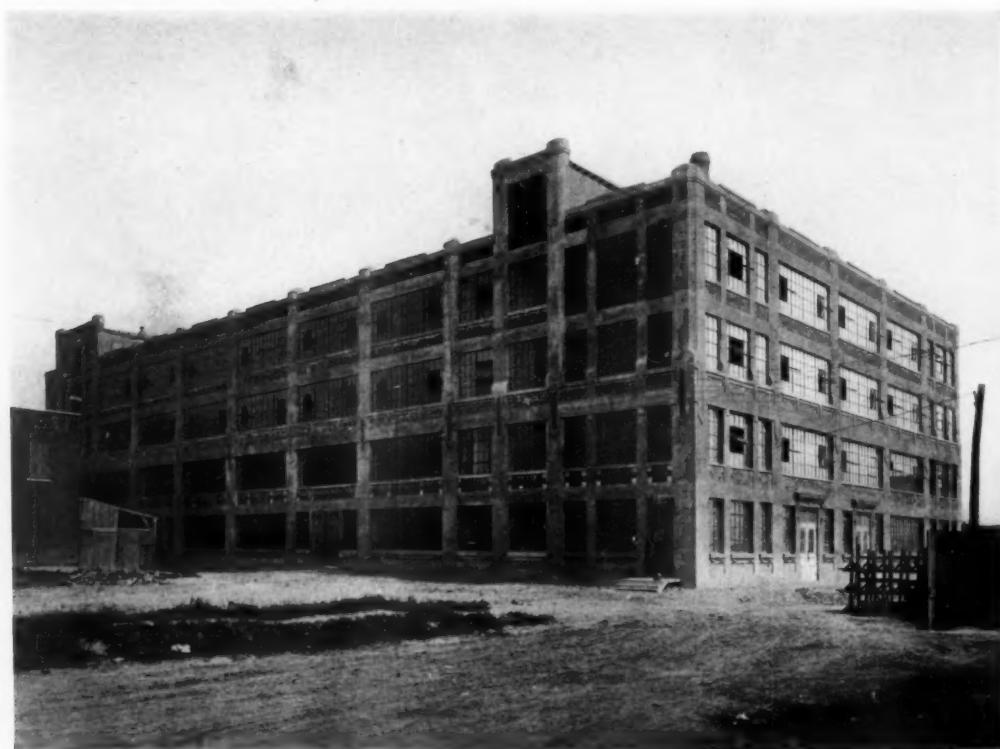
BUILDING OF THOMPSON & NORRIS CO., MONTREAL, CAN.
