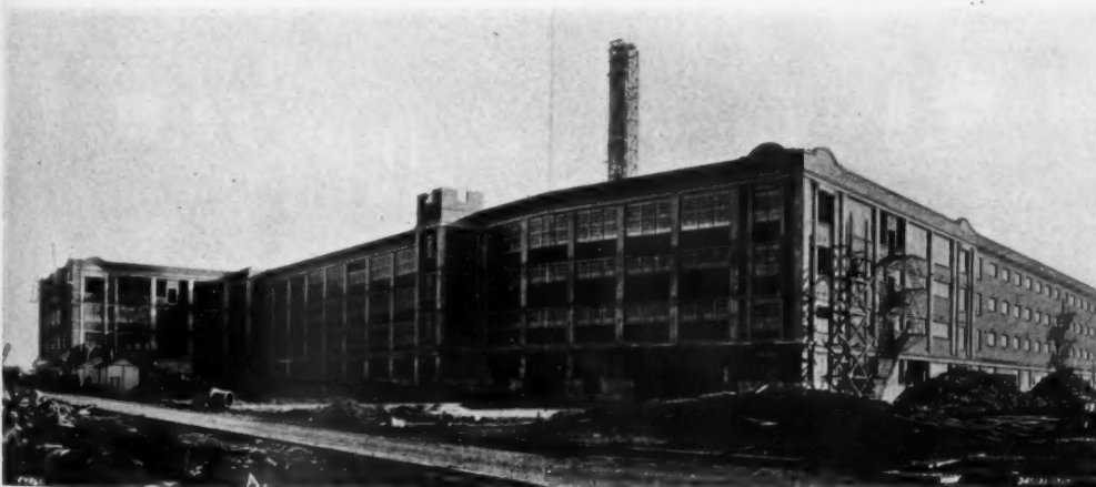
PROGRESS PHOTOGRAPH, DECEMBER 21, 1917
