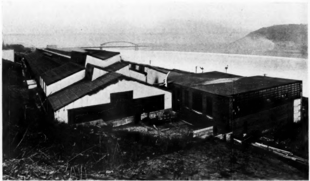
FORGE SHOP, HUBBARD & CO., PITTSBURGH, PA.
