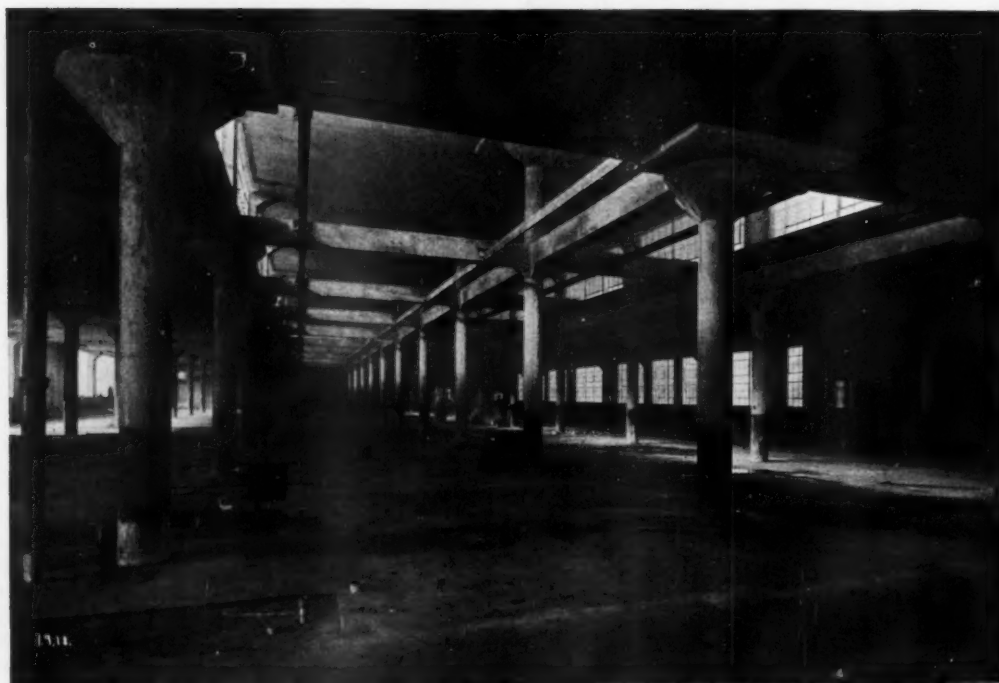
REINFORCED CONCRETE FACTORY SPACE, UNIT B
