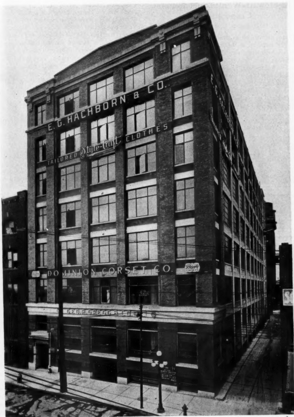
FACTORY BUILDING OF GEORGE R. GREGG CO., TORONTO, ONT., CANADA BERNARD H. PRACK, ARCHITECT
