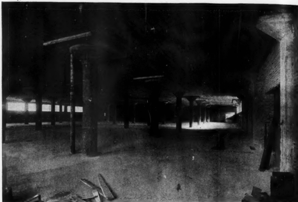
REINFORCED CONCRETE WAREHOUSE, UNIT B
