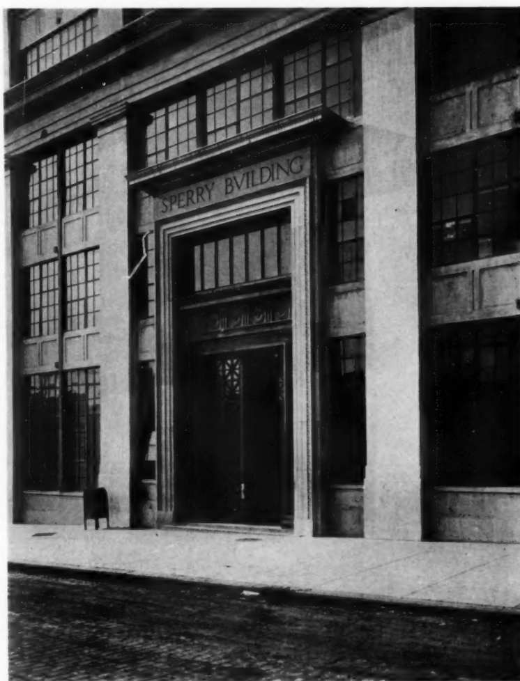
DETAIL OF MAIN ENTRANCE BUILDING FOR SPERRY GYROSCOPE CO., BROOKLYN, N. Y. HELMLE & CORBETT, ARCHITECTS
