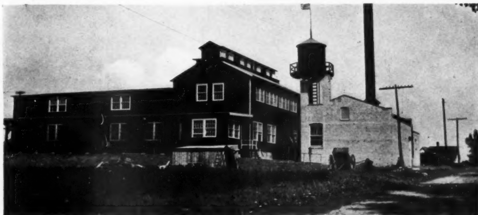
EATON, INDIANA, PLANT—REID MURDOCH & CO. GEORGE C. NIMMONS & CO., ARCHITECTS
