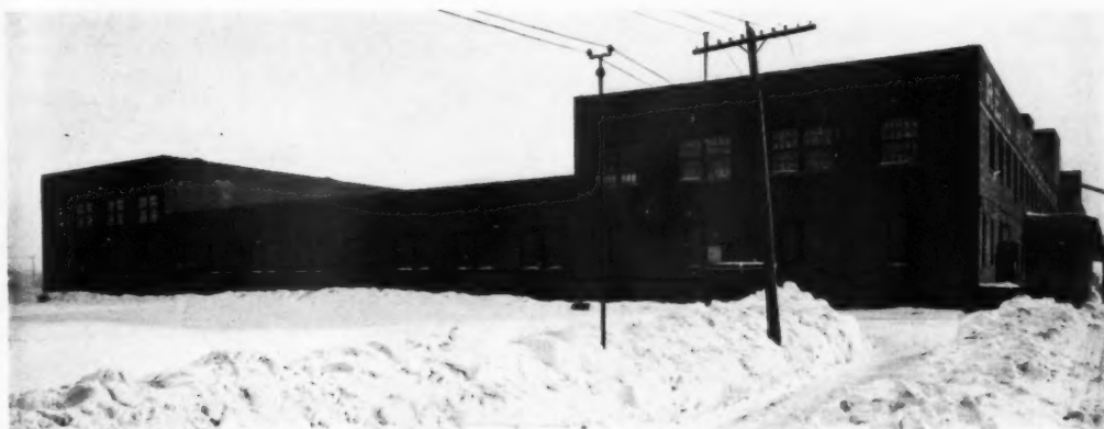
HAMMOND, INDIANA, PLANT—REID MURDOCH & CO. GEORGE C. NIMMONS & CO., ARCHITECTS
