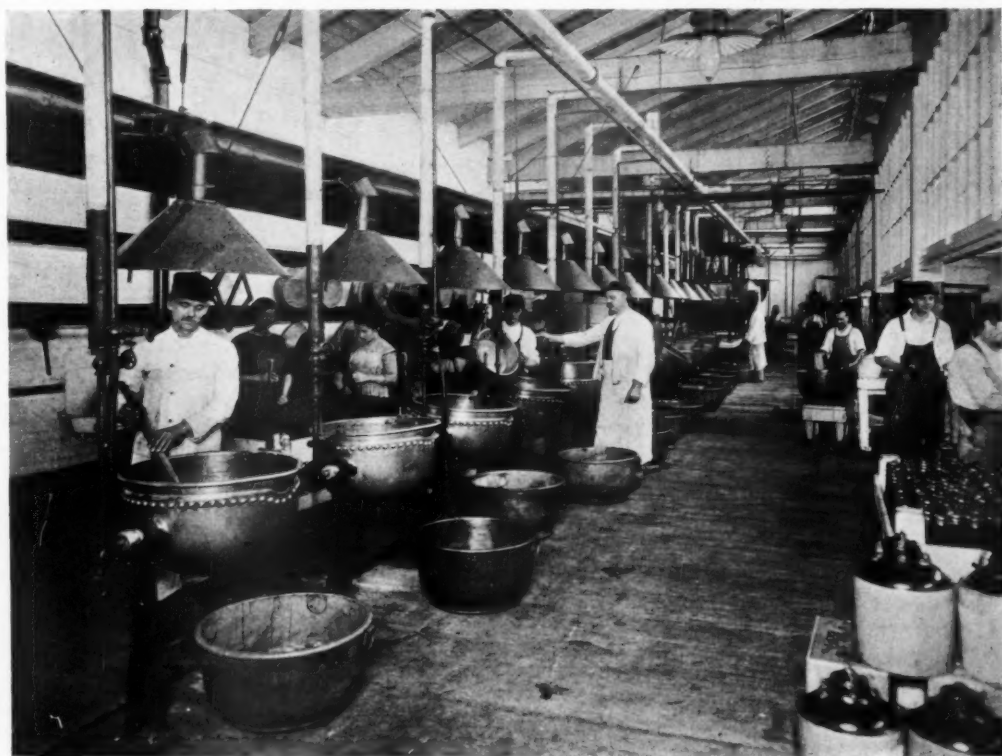
PROCESS ROOM, SHOWING COOKING KETTLES HAMMOND, INDIANA, PLANT—REID MURDOCH & CO. GEORGE C. NIMMONS & CO., ARCHITECTS
