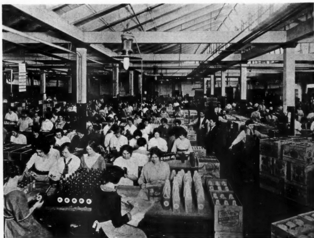
LABELING AND PACKING ROOM HAMMOND, INDIANA, PLANT—REID MURDOCH & CO. GEORGE C. NIMMONS & CO., ARCHITECTS
