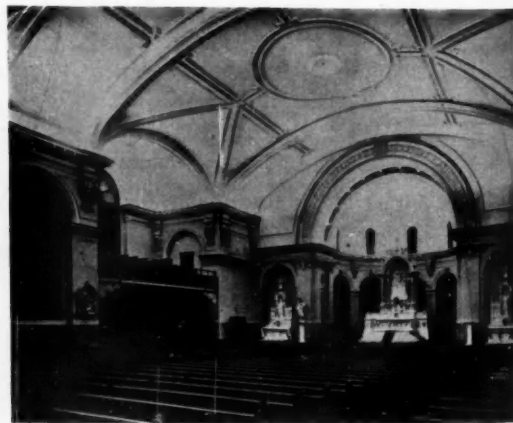
Fig. 2.—The "quantity" of light and the "efficiency" of obtaining it from ceiling reflection are insignificant details compared with the individual opinion of the architect regarding the effectiveness of ceiling brightness as a revealing agent. In Fig. 1 the ceiling is revealed by light directed upward from the floor. In this picture supplemental cove lighting discloses one phase of detail and ornament, evidently in accord with the architect's sentiment. The ceiling diffusing plate has been used here as in Fig. 1, and that sufficient light obtains is evidenced by the brightness of the top of the pew-backs.
