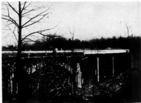
CONSTRUCTION VIEW, SHOWING ARCH SPAN DECK FALSEWORK
