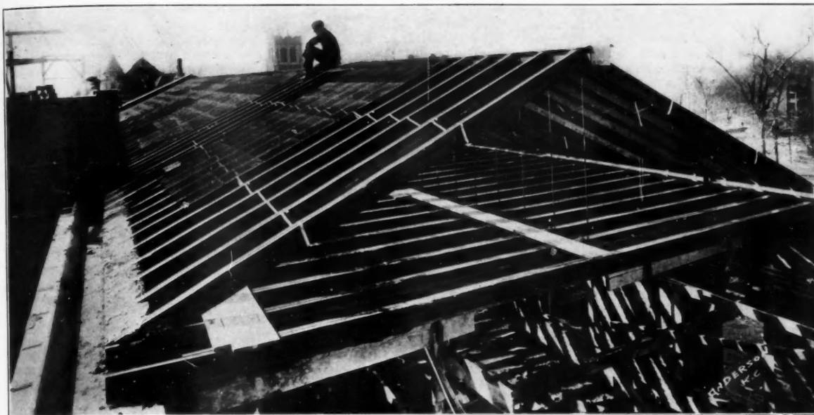
Pressed steel sections, used here in the same way as wood rafters, show the universal adaptability of Berger's Metal Lumber. The building is Mercy Hospital, Kansas City, Mo. Geo. A. Fuller Const. Co., General Contractors.
