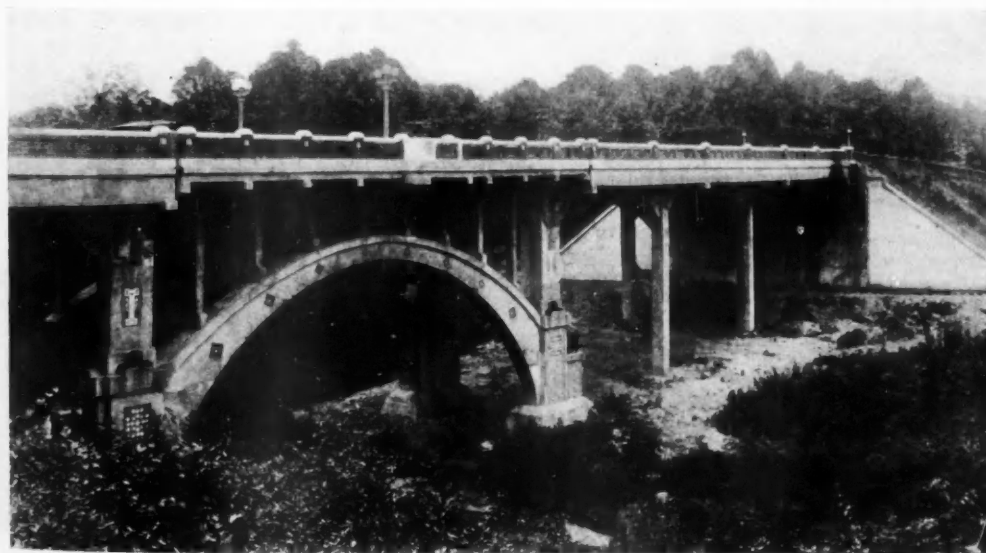
PIEDMONT PARK BOULEVARD BRIDGE, ATLANTA, GA.
